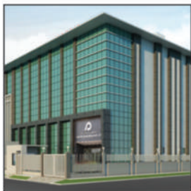
B-14, Sec. 80, Noida P.T.M.T. Taps, Seat Covers, Concealed Cisterns, Ball Cocks, Cabinets, Soap Dispensers, Garden Hose Pipes, Connection Hose Pipes, Corner Shelves, Floor Gratings
