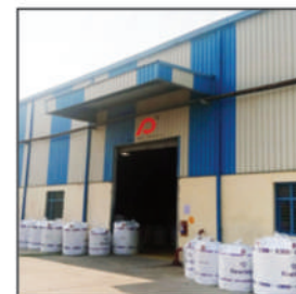
Plot-81, Sec Ecotech-1, Extension, Greater Noida Water Tanks
